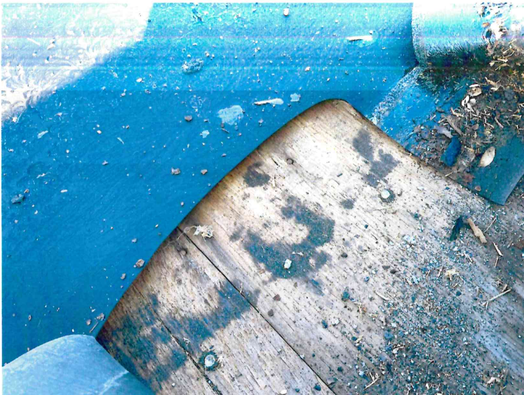
Rubber roofing over plywood
